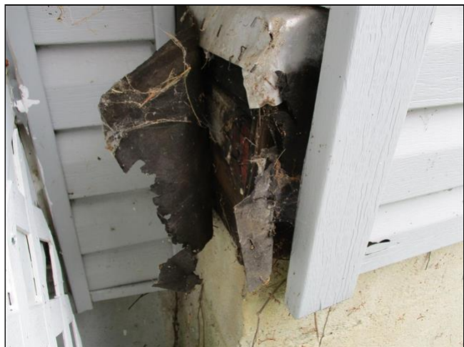
A. Item 2 Missing siding at pantry bump-out
