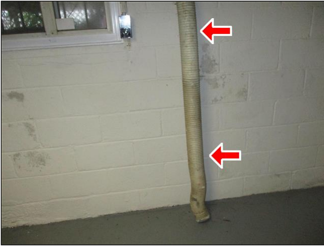
K. Item 1 Unsafe plastic dryer vent
